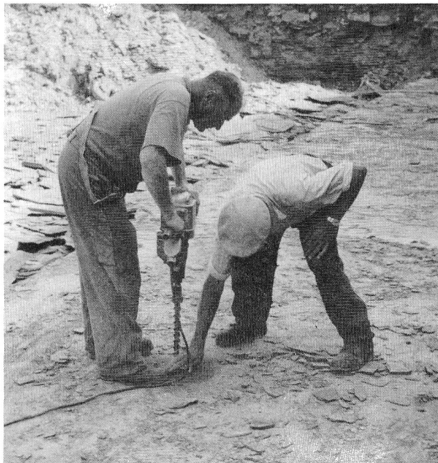
Fig.5. Boring a blasting hole in the Unteren Schiefer, just above the Fleins, in the quarry of J. Fischer, Ohmden, 1968. Blasting loosens the rock before extraction.
