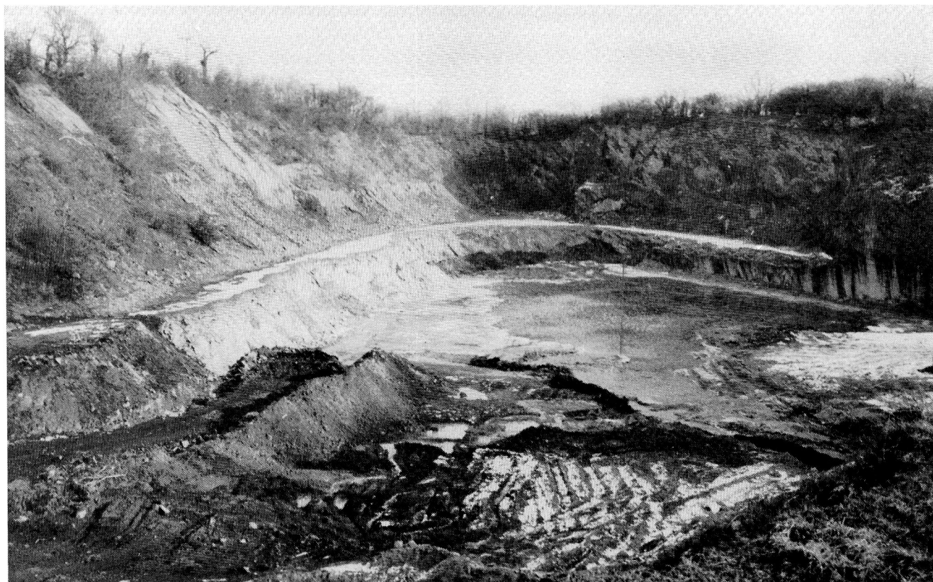
Fig.3. Coplow Quarry at the start of infilling work, photographed 11 February 1986. The terrace marks the top of the old water-level.
