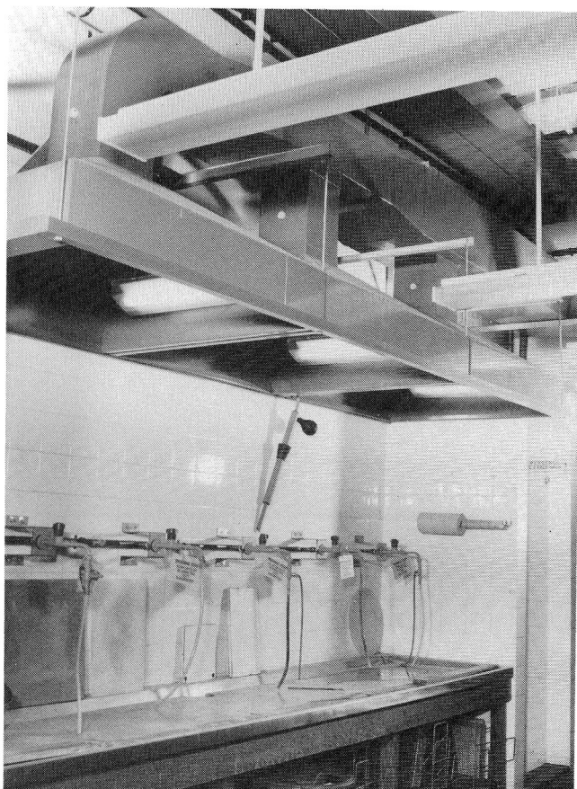
Fig.4. Canopy hood arrangement. Palaeontology Laboratory, British Museum (Natural History).
