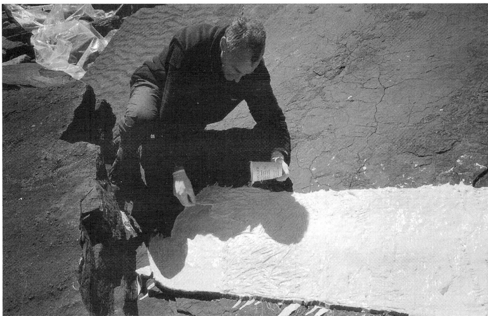
Figure 3. Applying the second coat of silicone rubber.
