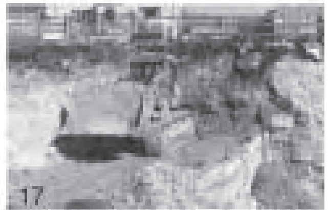
Figure 12. In the foreground, volunteers are marking the blocks and the fractures onto a plan and the pavement at Townsend Road, to allow reassembly.
