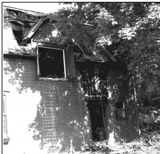
Figure 1. Side view of the barn showing the external door to the workroom where the fire started. The charred clapboard shows where the fire flared upward when the door was broken open and ignited the roof through the soffit vents under the eaves. Destroyed portions of the roof are visible, but the dormer holding the hay doors was untouched by the fire.
