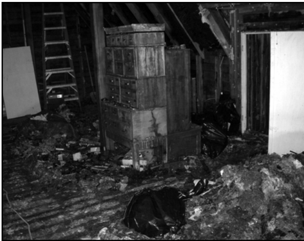
Figure 4. Much of the second floor was covered with debris consisting of mineral specimens, labels, wet cardboard, wet fiber glass insulation, roofing shingles, burned rafter fragments, fused insulation, and wet plasterboard. A path to the hay doors on the right has been cleared, and my sorting of specimens from the debris has begun. To the left is the "Slough of Despond" and to the right is "Mount Manlius." Note the remaining two oak cabinets. The finish on both was ruined. The shorter cabinet on the left was a total loss because swelling buckled the drawer fronts and bottoms. The taller cabinet was intact and could be refinished.
