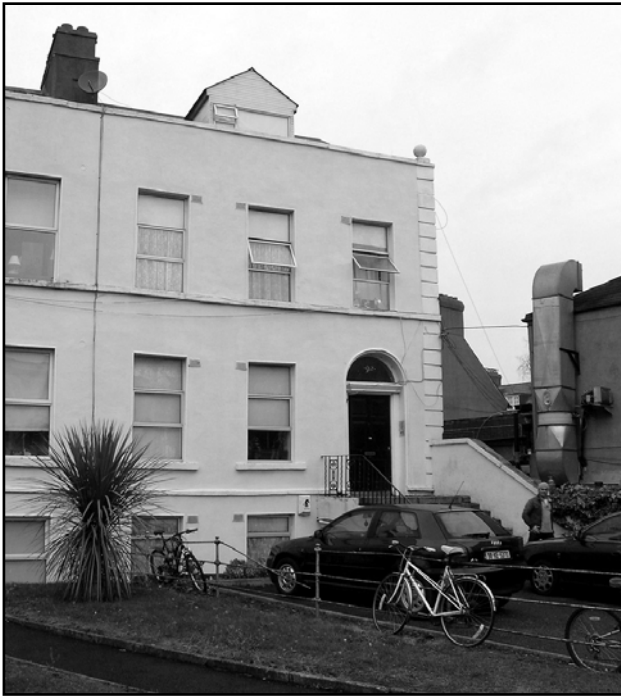
Figure 18. "Apsley Lodge", 92 Rathgar Road, Rathgar where Baily lived 1872-81.
