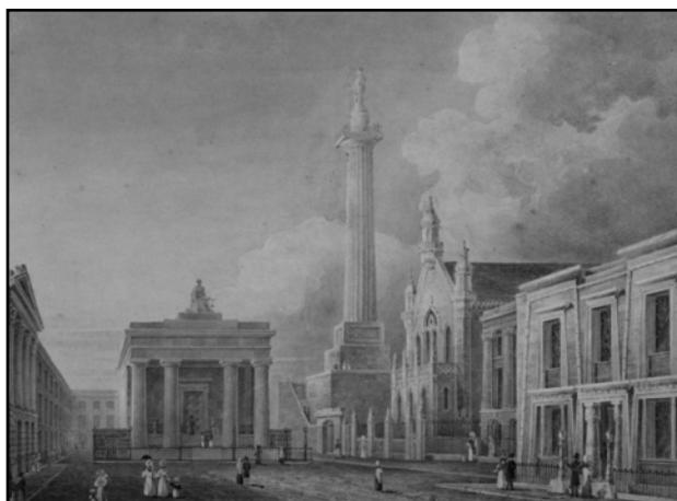
Figure 5. The Civil and Military Library in Devonport, Plymouth City Museum and Art Gallery ©. It is the closest building on the right and was designed to look like an Egyptian Temple
