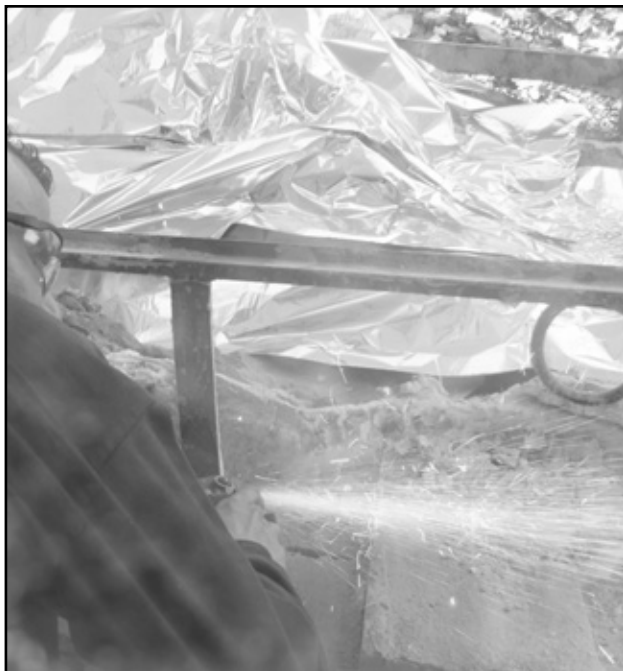
Figure 11. Cutting the metallic reinforcement.
