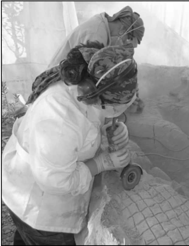
Figure 7. Cutting the matrix with a small radial saw.
