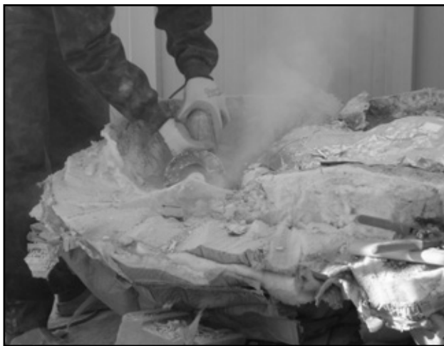
Figure 10. Cutting the resin and fibreglass binding.
