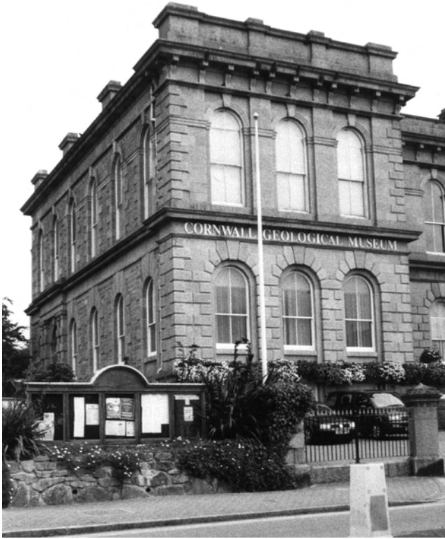
Figure 2. Premises of the Royal Geological Society of Cornwall, St John's Hall, Penzance, built for the Society in 1868, and now known as the Cornwall Geological Museum. Photographed by David Freeman, July 2002.
