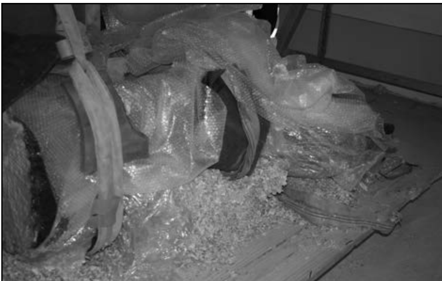
Figure 7. Channels excavated through the compressed sawdust allowing lifting slings to be fitted.
