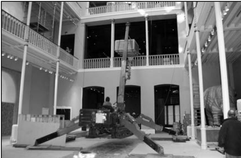
Figure 9. Spider crane lifting crated geode from Level 1 to Level 3.
