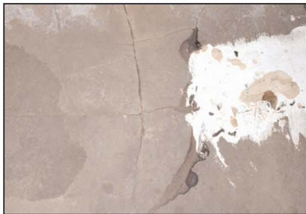
Figure 3. Detail of damage to underside of inlay panel.
