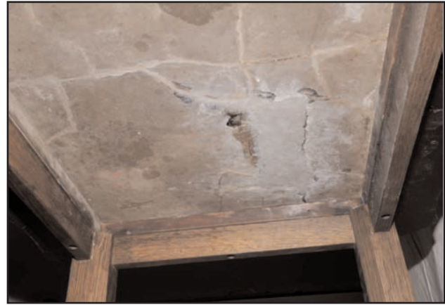
Figure 5. Detail of underside after conservation.
