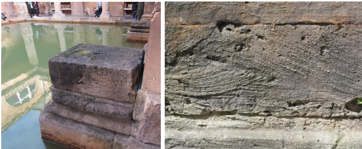
Stone at the Roman Baths, Bath: a) the base of a Roman column with a bolt-hole cut into the top; b) a block of Roman stone with cross-bedding and burrows.
